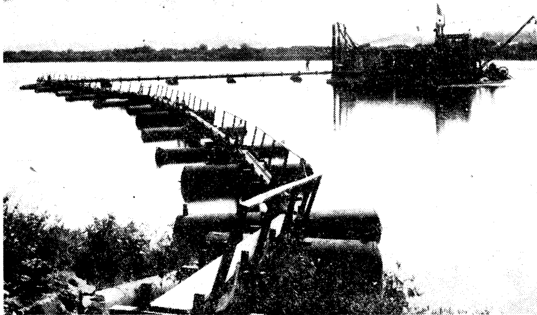
Electric power dredge pumping silt and mud out of the Torresdale basin through 15-inch steel pipe to basin on low lying land
