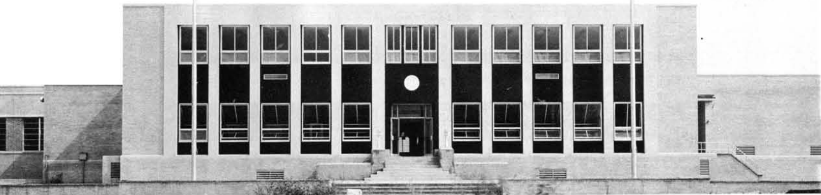
Filter building: Attractive and modern is the four and one-half acre filter building which houses offices, laboratories and 94 rapid sand filter beds.
