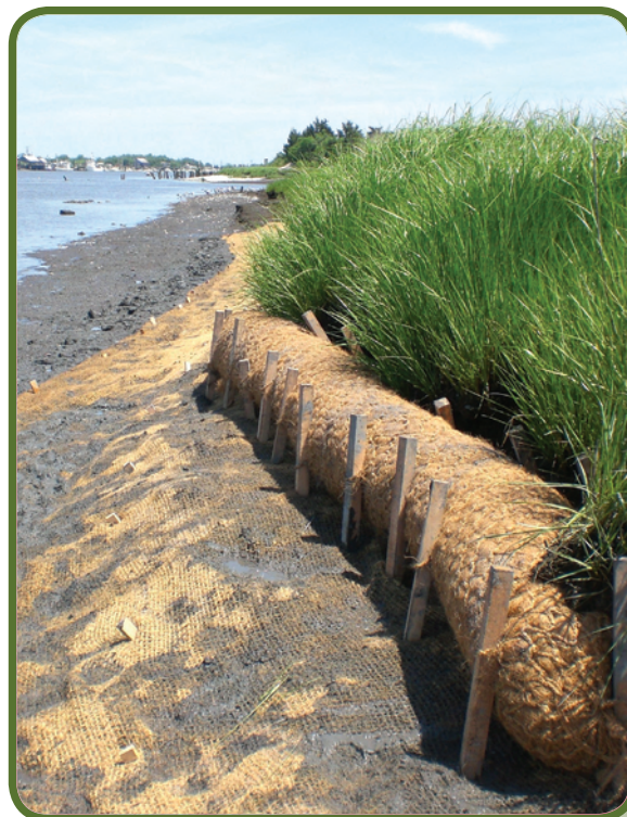
A coconut fiber log is deployed along the edge of a tidal marsh in Bivalve, New Jersey, in an effort to establish a "living-shoreline" reef that may soon protect against erosion.
