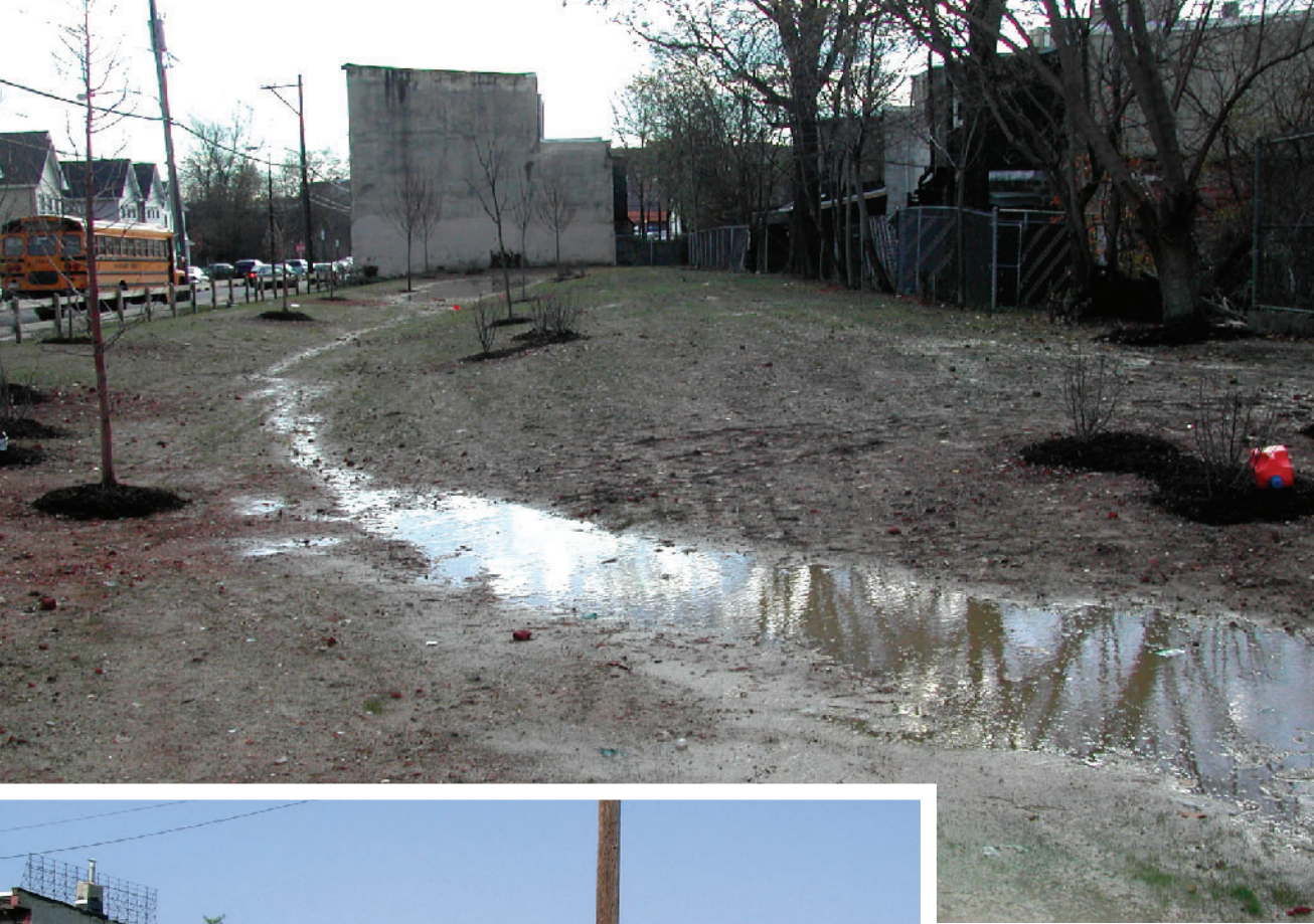
Top: Trenches and berms harness rainfall on the sites, where it is slowly absorbed back into the ground over a 24- to 36-hour period.
