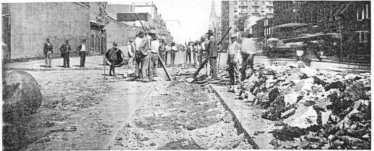
PRELIMINARY WORK IN PIPE LAYING, removing asphalt surface and starting trench.
