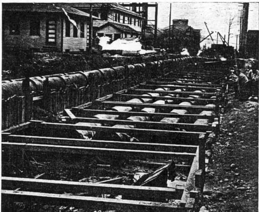
Giant Pumping Mains from Lardner's Point; four of 60-inch diameter, one of 48-inch diameter, one of 30-inch diameter; combined, these six pipes have a daily capacity of 300,000,000 gallons of water
