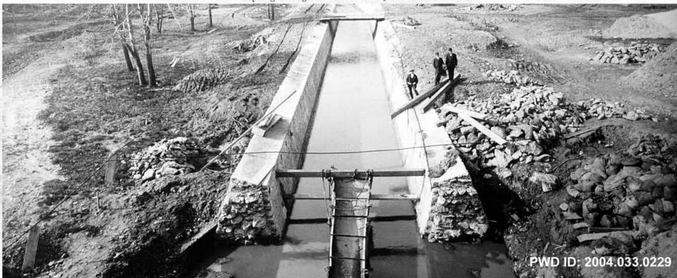
WINGOHOCKING SEWER SYSTEM on Annsbury Street; 14.8 miles in length; when completed it will be 16.11 miles in length; built of brick; diameter 17 feet 6 inches; will be 20 feet in diameter at outlet into Frankford Creek when completed. This sewer system serves one of the most important sections of the City, emptying into the Frankford Creek at Wingohocking Street and carrying sewage for the northwestern district as far as Chestnut Hill, altogether serving a district of 5,500 acres, largest drainage area in City.
