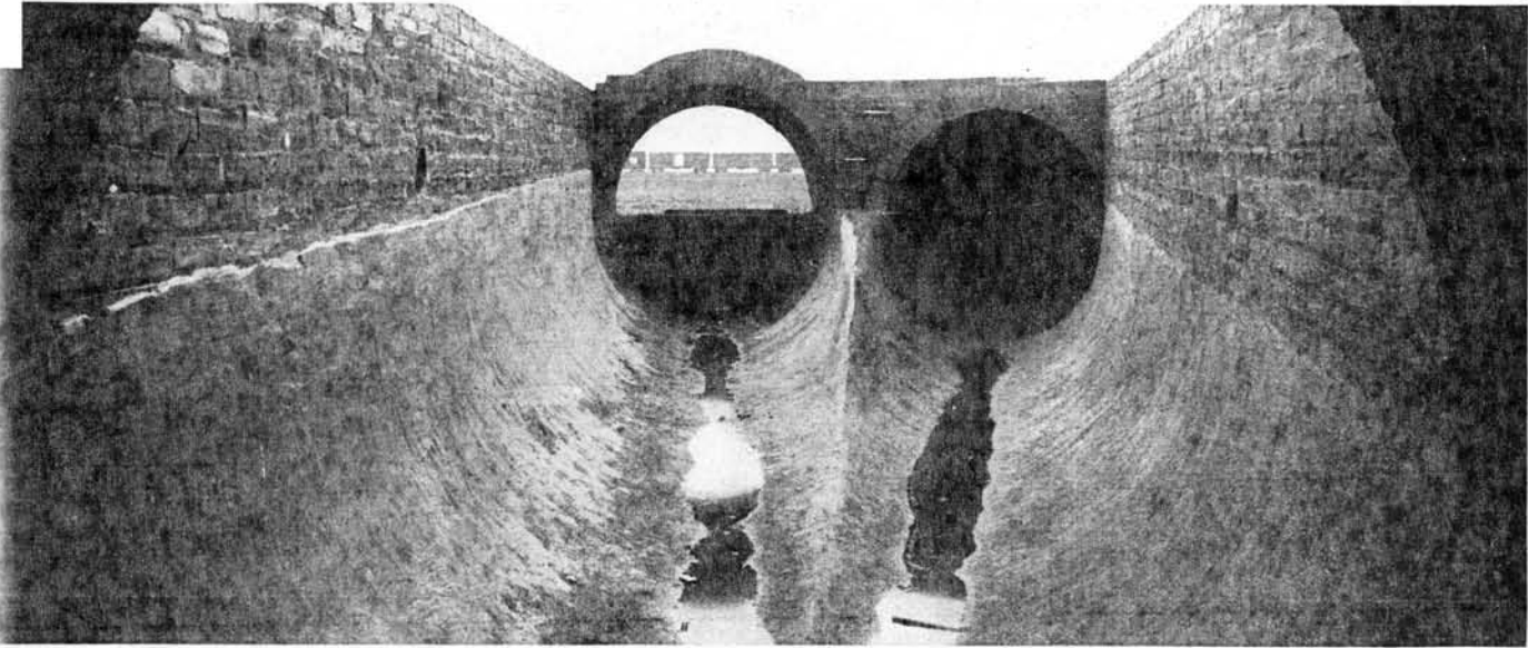
FUNCTION CHAMBER OF SEWER SHUNK AND FRONT STREETS, where two six-foot six-inch sewers run into a seven-foot six-inch sewer. This sewer is two and one-third miles in length, and built of brick.
