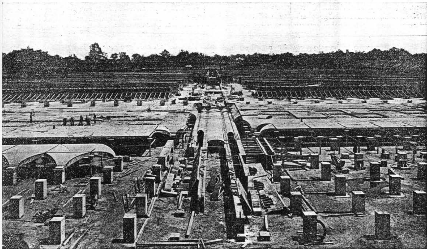
QUEEN LANE FILTER PLANT now nearing completion. This new filter is built in one section of the Queen Lane Reservoir. The plant is a two-story structure. Filtered water basins occupy entire space under final filters, such space being 1,056 feet by 709 feet; when filled to its normal depth, nine feet, it will have daily filter capacity of 75,000,000 gallons. The floor of the original reservoir forms the floor of the new filtered water basin.
