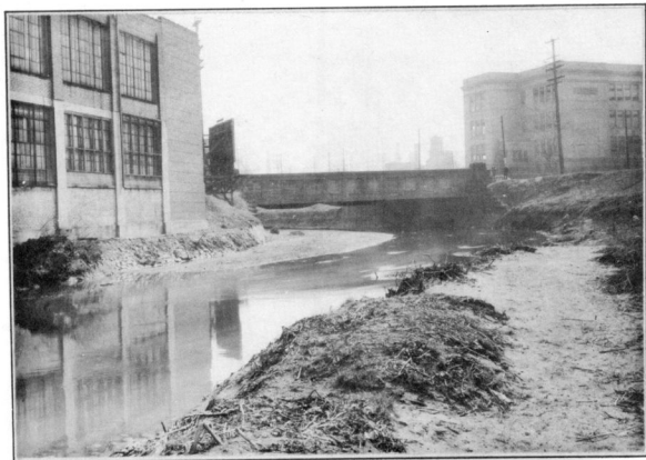
B- LOOKING DOWNSTREAM AT TORRESDALE AVENUE BRIDGE. LOWER SECTION OF WIN- DOWS AT LEFT FILLED IN TO PREVENT FLOOD DAMAGE.
