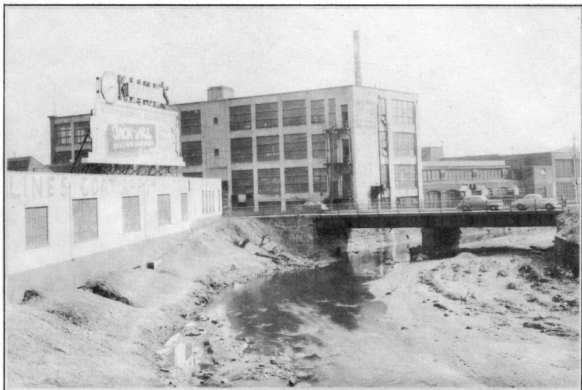
A—LOOKING DOWNSTREAM AT WORRELL STREET BRIDGE. PROPOSED IMPROVEMENTS WILL REQUIRE REMOVAL OR REPLACEMENT OF THIS BRIDGE.
