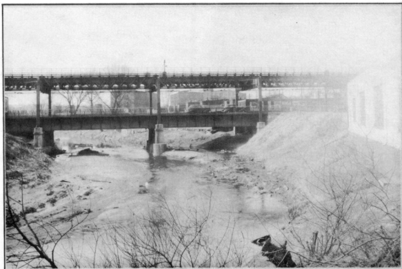
B—LOOKING UPSTREAM AT KENSINGTON AVENUE BRIDGE. CENTER LINE OF PROPOSED CHANNEL IS LOCATED IN LEFT HAND OPENING.
