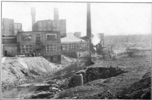
A —LOOKING DOWNSTREAM FROM BRISTOL STREET EXTENDED. ENCROACHMENTS ON LEFT BANK HAVE FORCED CREEK TO ERODE RIGHT BANK.
