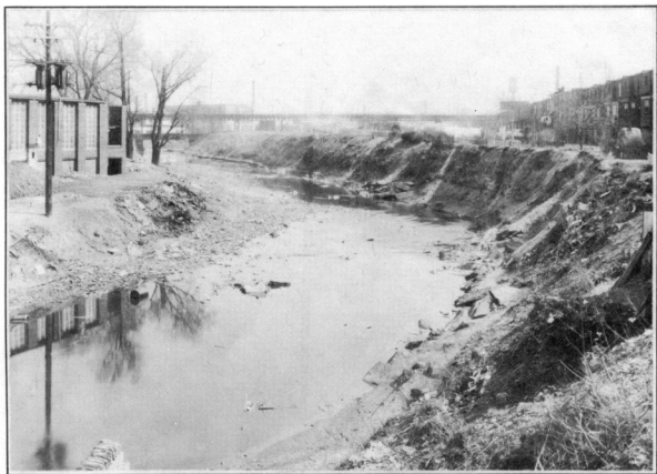
B - LOOKING DOWNSTREAM FROM LEIPER STREET TOWARDS KENSINGTON AVENUE. PROTECTION OF BANKS AT RIGHT REQUIRES HIGH WALLS OR A SECTION OF COVERED CONDUIT.
