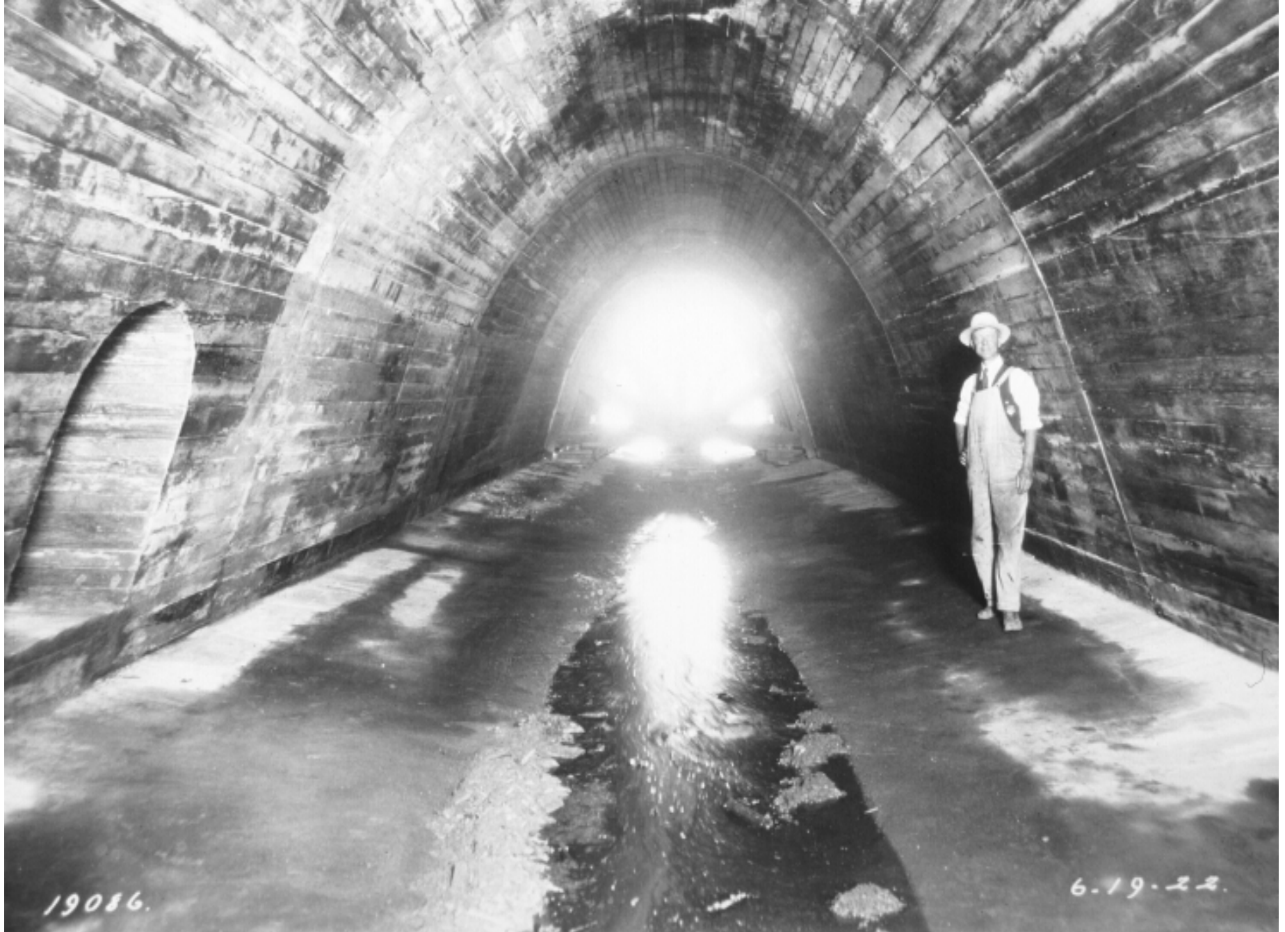
Rock Run Sewer in Ashdale Street, 1922
