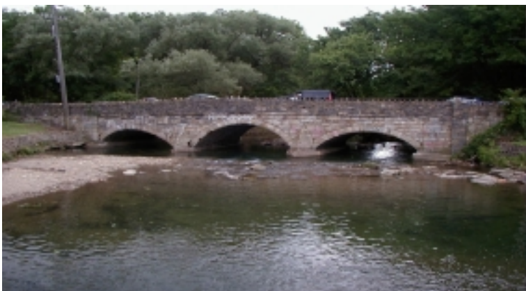
Adam's Avenue at Crescentville Road after the Waterways Restoration Team clean up
