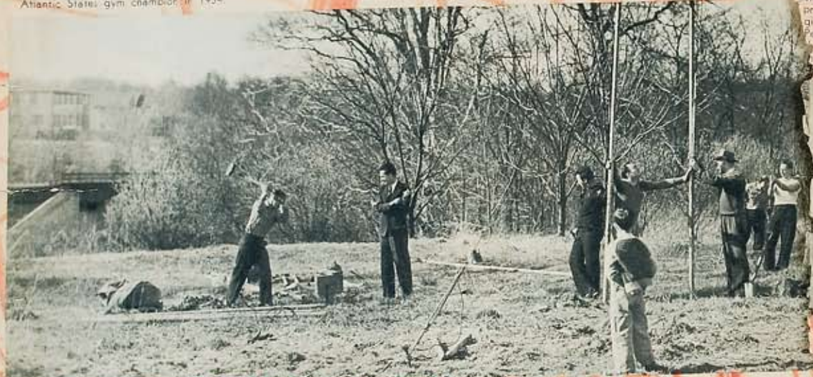
Erection of the 32-foot trapeze rigging presented some problems. Greatest was uneven ground, another was the replacement of old rope, as the equipment had been in storage for the last five years while the boys were in service. Supports are of steel tubing made up in sections for pitman lining.
