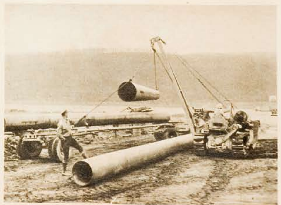
Oil will soon flow through these sections of the "Big Inch" pipeline, shown ready to be put into the trench blasted out of the river bed. Immediately after the blast drilling was resumed for additional explosions.
