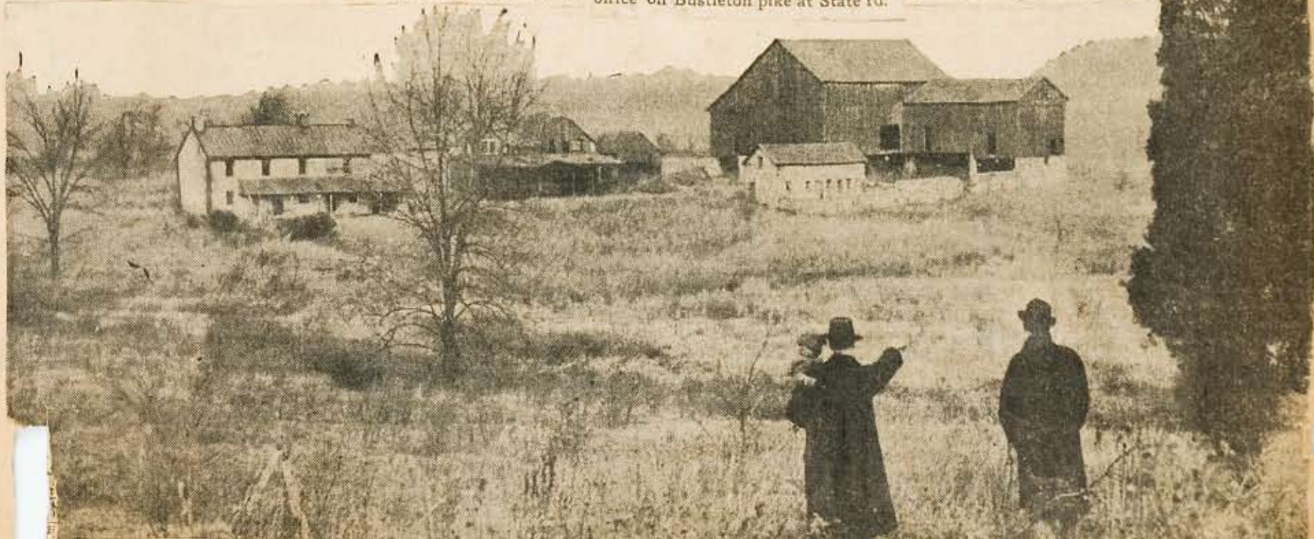
From the "Hill of Vision," two members of Bryn Gweled Homesteads see neat homes and carefully tended gardens replacing the weeds and brambles of the 238-acre estate on Stump Bridge rd. near Feasterville. Buildings in the foreground will be reconstructed as a community center.
