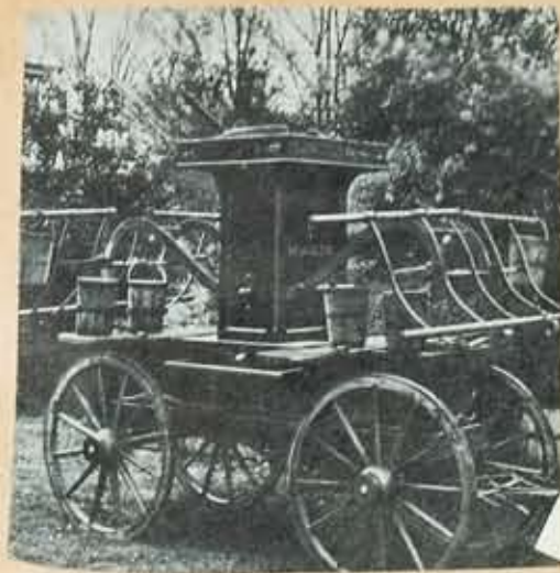
Newtown is justly proud of an efficient volunteer fire company, originally the Washington Fire Company organized in 1824. Their first engine was built by Patrick Lyon of Philadelphia in 1796.
