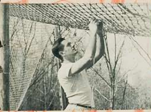
Constant repairs are needed on the safety net. It is inspected every time used, and here, Frank Longbottom, 1328 Howell st., gives a repair. Nets are handmade and may last for 20 years.
