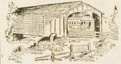
OLD "DUMMY" BRIDGE Over Frankford Creek.
