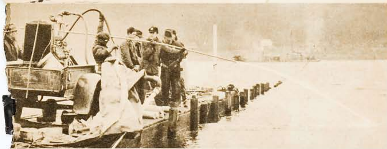
Three weeks were required to prepare for the blast. Here, explosive experts lower dynamite into steel containers which have been drilled into the river bed. In the background is the proposed path of the pipeline across the river.
