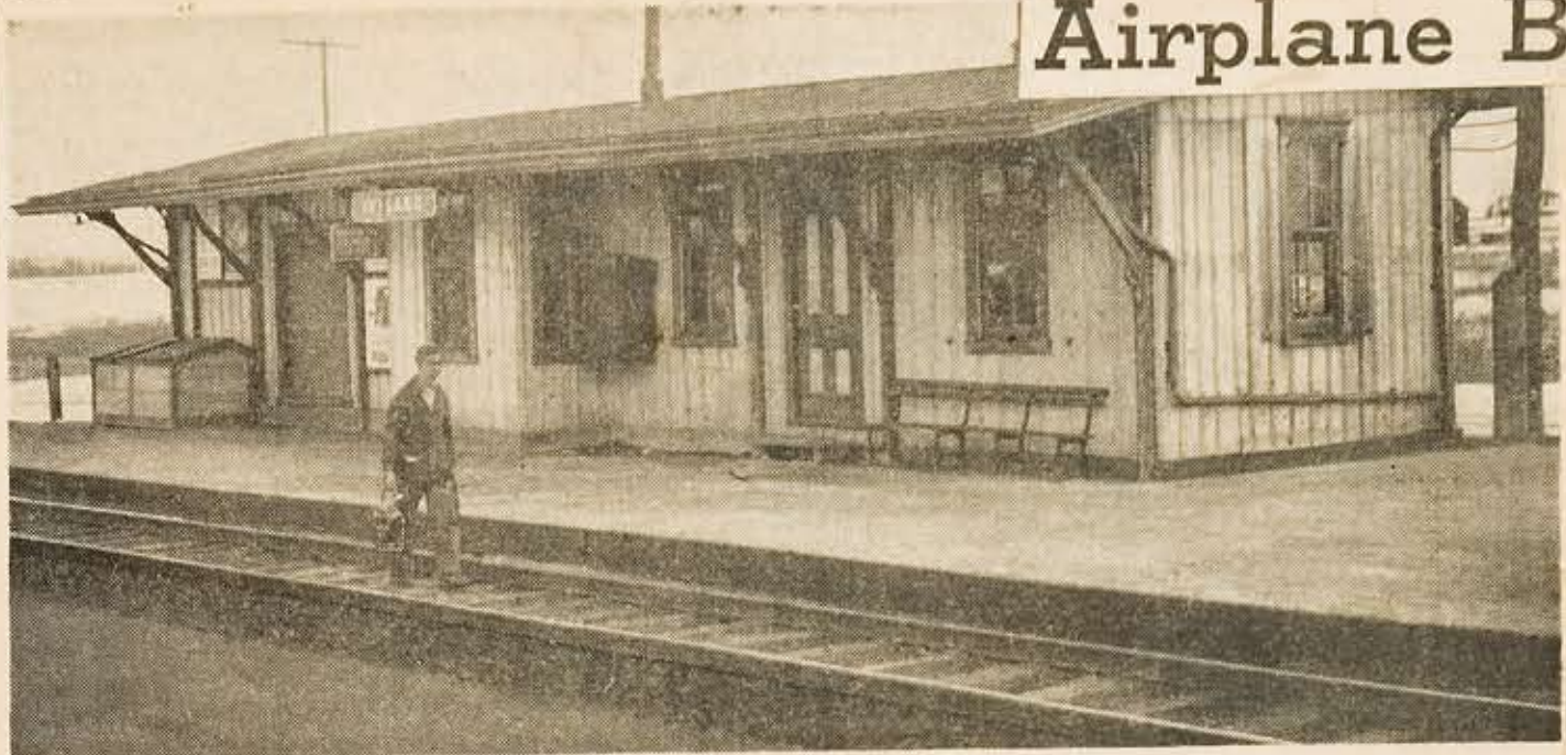
Residents of Ivyland hope this railroad station will be replaced by a modern structure if expected town prosperity results in more traffic
