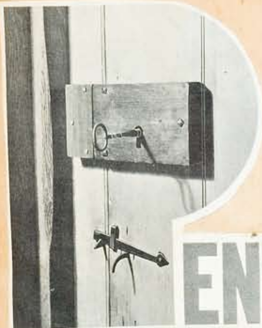
1—Some hardware of the period has been found and used; other hinges, locks, latches and keys are faithful reproductions, as this safeguard of the old brew house at Pennsbury.
