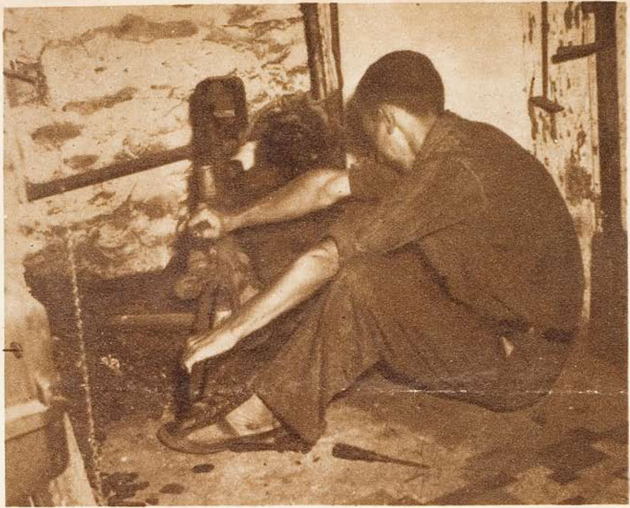
Depressions don't bother Point Pleasant workmen. They shift from one trade to another with alacrity. G. Walton Howarth, town electrician, takes on a plumbing job. He also is a carpenter.
