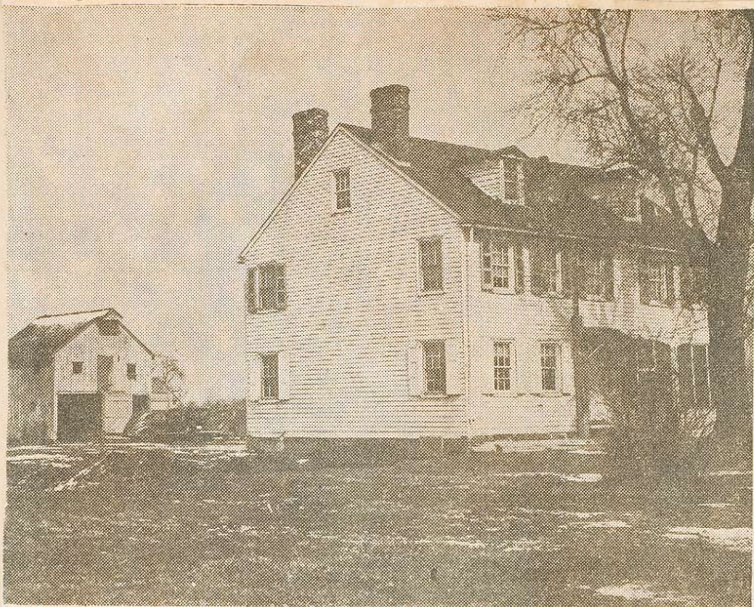
This house, occupied now by caretaker of estate along Delaware, will be moved aside. It rests on original foundations of Penn's home, which will be entirely rebuilt
