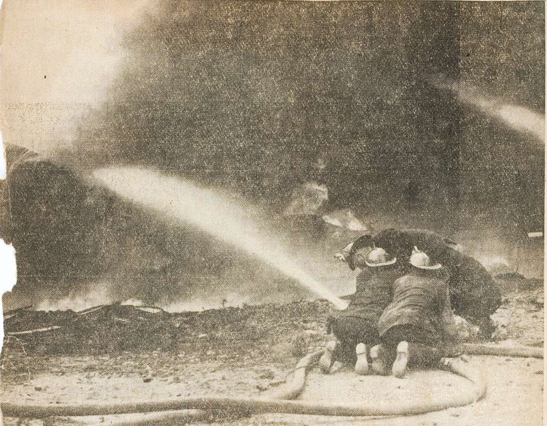
Two firemen handle one hose line in an effort to beat out fire in the foundations of the export shed at the Tiona Petroleum Company plant, Tulip and Wyngate sts., where a four-alarm blaze destroyed thousands
