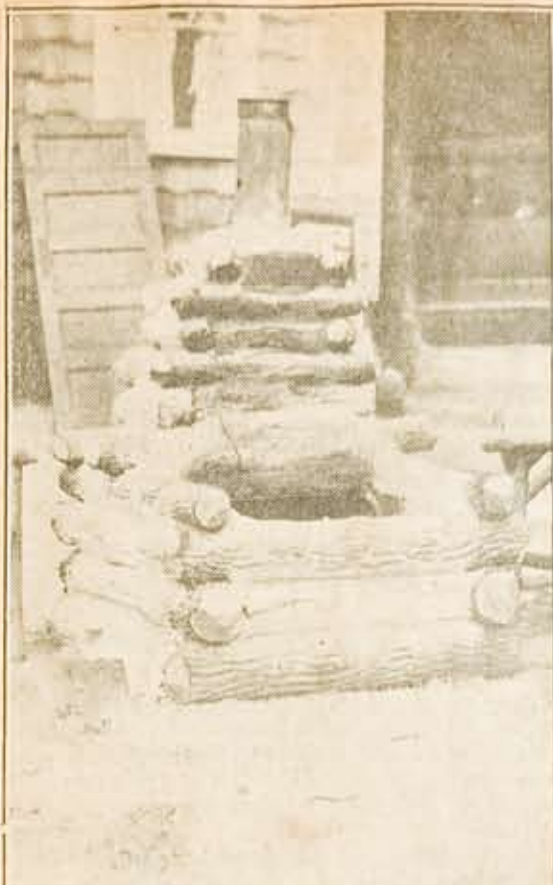
A Rustic Fireplace, built by William H. Crump, near the cabin in which he lives, on Ashton road, West Torredale. It is 45 inches square and built of logs and clay. The design was copied from pictures Mr. Crump saw in a book about the Civil War. Sassafras logs were employed and the firebed lined with tin cut from a receptacle salvaged in the neighborhood. The smokepipe was likewise a discard. After the logs are set together with clay, a slow fire must be lighted and kept burning until the clay has hardened.
