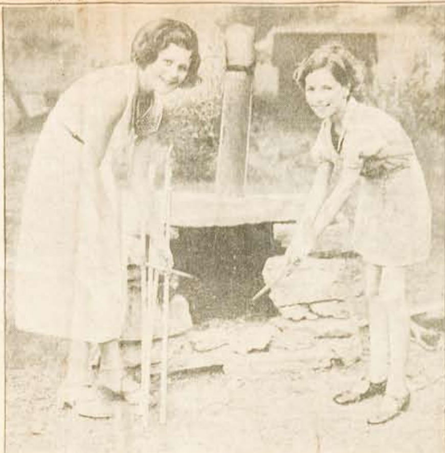
Old Stones from an Abandoned Greenhouse, clay from a nearby creek, and a piece of discarded sheet metal were the materials used to make a fireplace for Louis Moss, on Ashton road, Torredale. His grandson, Stanley Kaufman, was designer and builder. The firebed is directly on the ground. And the family discovered a use for discarded miniature golf clubs. The club-heads were removed, holes bored in the wood and forks stripped of their own handles fitted into the golf sticks. Perfect for toasting marshmallows! In the picture Estelle Moss (left) and Anna Schleincofer show you how it's done.
