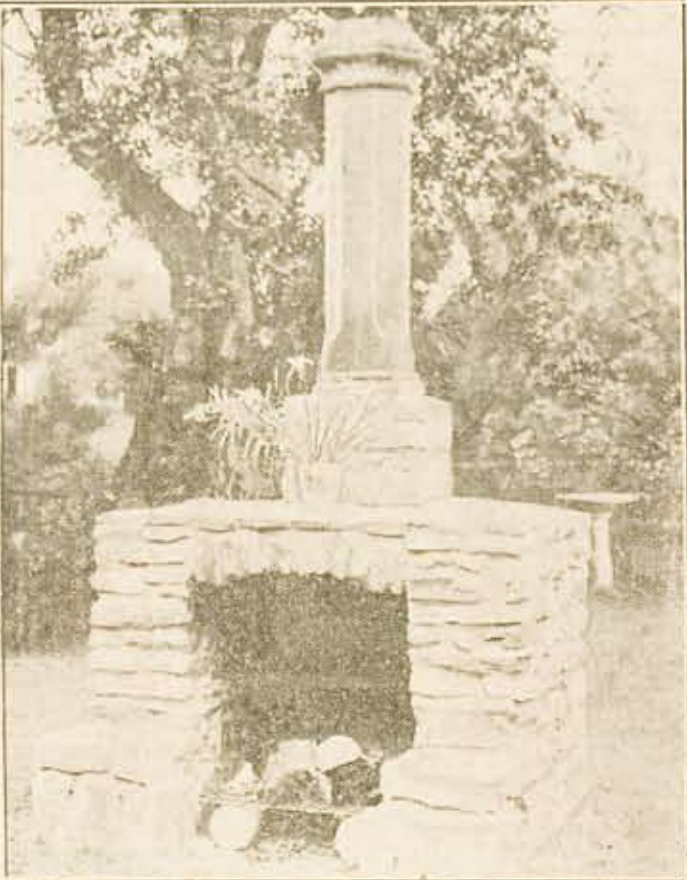
Of Stone and Cement with Copper Smoke Pipe at home of Mr. and Mrs. Allen Davis, Ashton road, Torredale, built in a day and a half by the neighborhood "handy man." A 16-inch base of cinders was thoroughly tamped before the 16-inch walls of stone and cement were set, with an arch shaped over a wooden frame. The fireplace is 5 feet, 5 inches wide, 60 inches deep, 12 feet high at the stack, with an oven space 45 inches square provided with iron rods and hooks for cooking. "Steps" in the stones at front allow space for cooking utensils. Black wire netting about the top of the pipe keeps sparks from flying.
