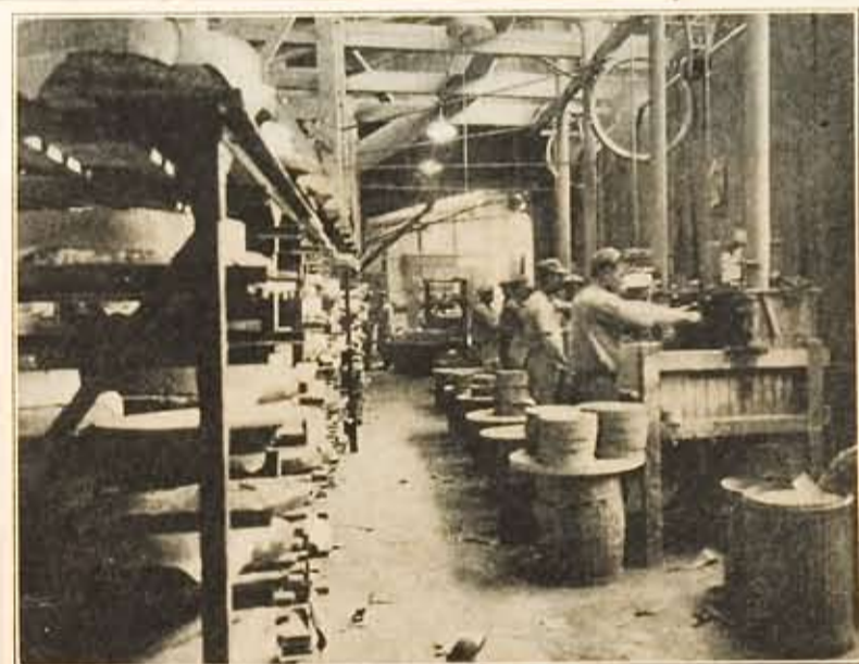
FIG. 3 — Shaving Department. Wheels being turned to approximate shape.
