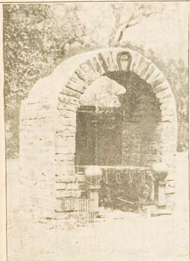
This Brick Fireplace on the Lawn of Isaac P. McGraw, Southampton road, Somerton, was built of bricks obtained when an historic old hotel was razed in Bustleton. The McGraw children dug a 12-inch pit with a foundation of cinders. Mr. McGraw set the bricks himself, using a wooden arch, with an opening at the back for draft. The grate is one discarded from the household furnace, and old cannon ball andirons support it. The top of the arch is adorned with a horseshoe. The McGraw family have turned out everything from broiled guinea hens to toothsome hot dogs.
