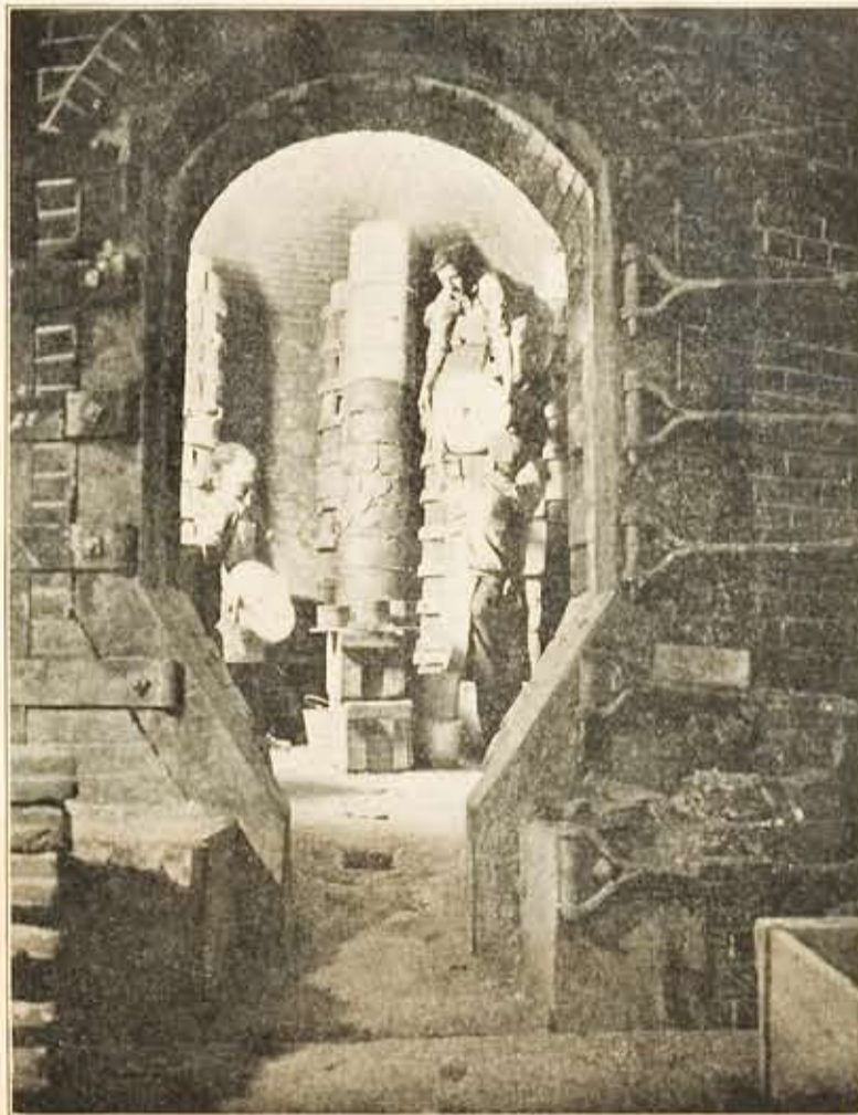
FIG. 1 — Setting a Kiln
