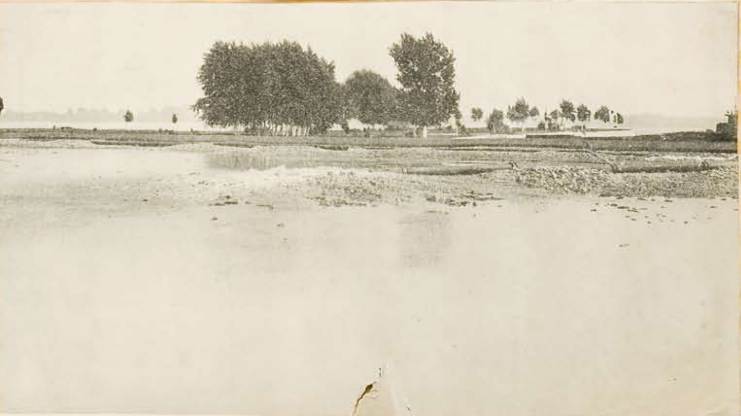
SECTION OF LOW LAND, LYING BETWEEN HOUSE OF CORRECTION AND DELAWARE RIVER, into which material raised by the dredge, whose operation is shown on page 6, is now being deposited. At this date when dredging was delivered to City, 25,000 cubic yards of earth have been removed from the Delaware River, shown in picture on opposite page, and the land located at this point and shown in this picture. There are 80 acres of such land located at this point and shown in this picture.
