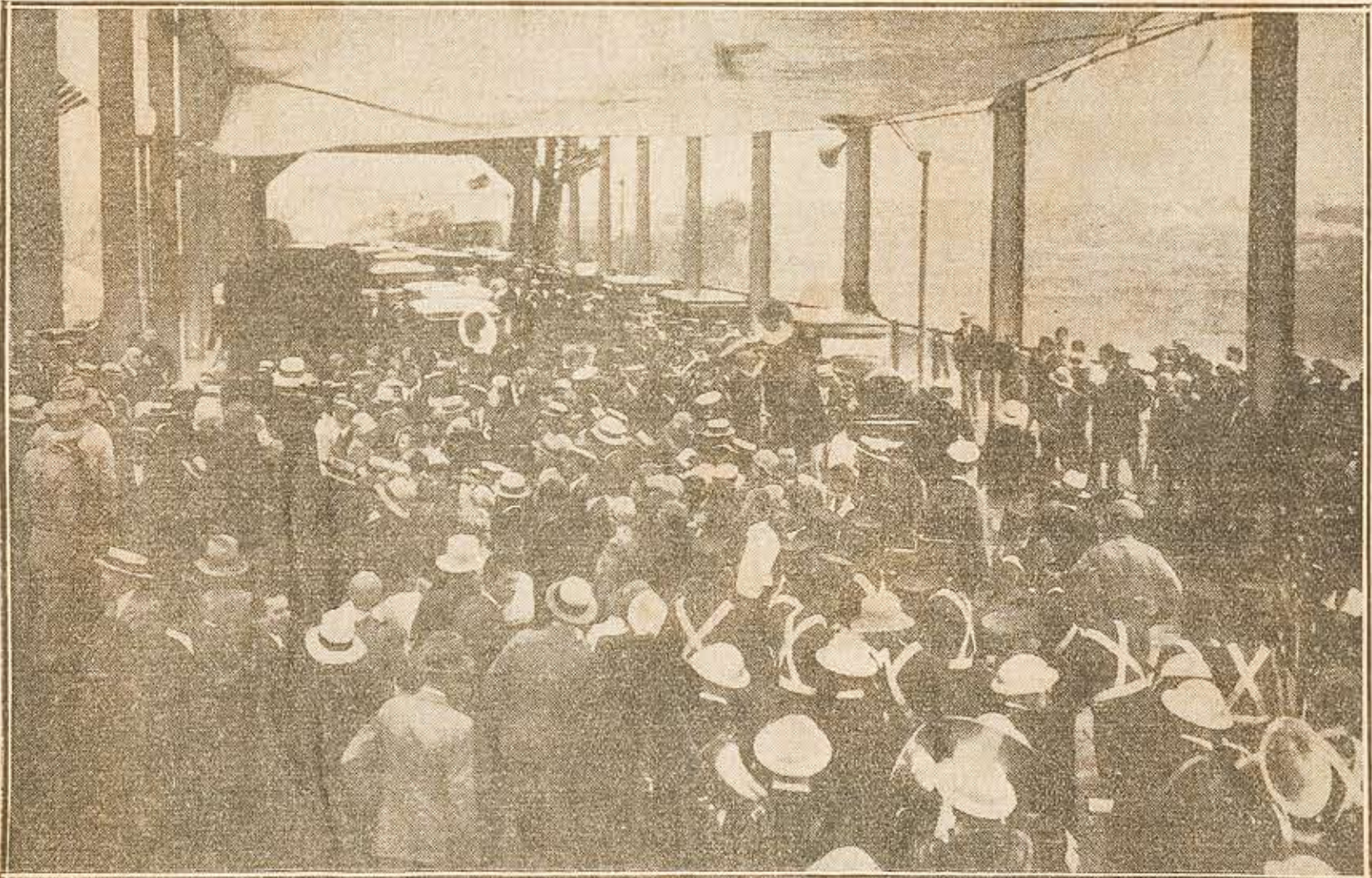
Ledge Photo CANVAS ROOF HASTILY ERECTED OVER CENTER SPAN OF NEW BRIDGE afforded some protection yesterday to a portion of the throng attending formal opening of Tacony-Palmyra span over the Delaware. Picture shows general view of crowd milling good naturedly while waiting for storm to let up enough to permit festivities to proceed. Notice how legionnaires, bandmen and other official participants are mixed up with unofficial but equally earnest bridge-openers
