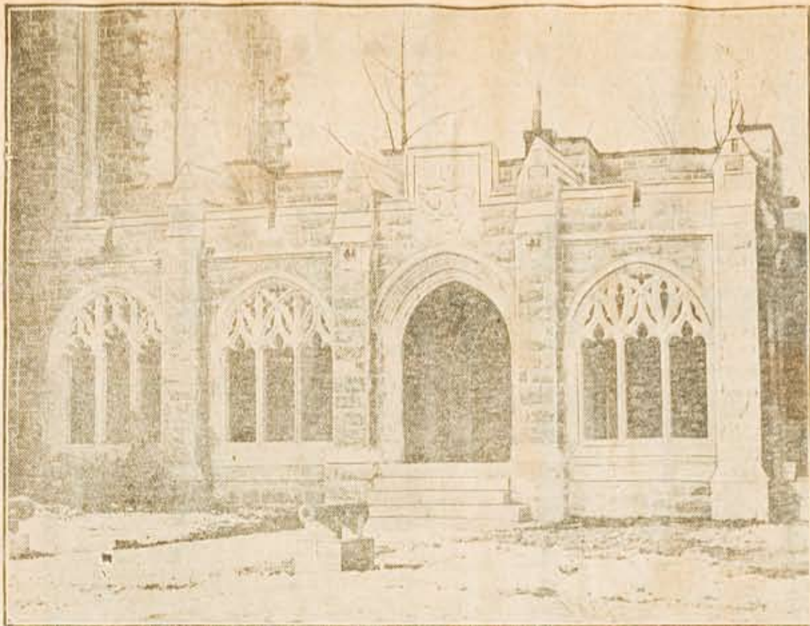
Porch of Allies Addition to the Washington Memorial Chapel at Valley Forge—It commemorates the Revolutionary services of Lafayette, DeKalb, Von Steuben and Rochambeau. The porch, built of Holmesburg granite and Indiana limestone, extends to the east of the Chapel along the south side of Patriots' Hall. It will connect the Chapel with the Robert Morris National Memorial Tower, which the Bankers of America plan to erect in honor of Philadelphia's Colonial financier. Revolutionary cannon are mounted in front of the porch.
